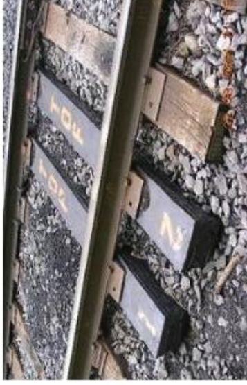
Two ties on a 3 degree curve with standard tie plates and rail spikes.
