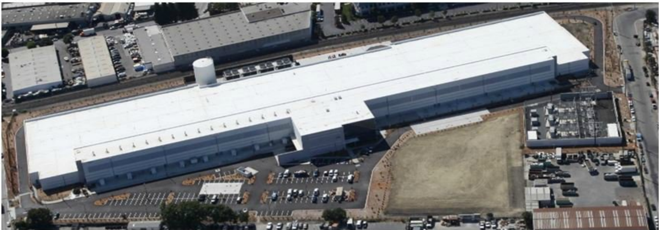
SCI Data Center - Santa Clara, CA
